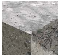
Steel fiber concrete
