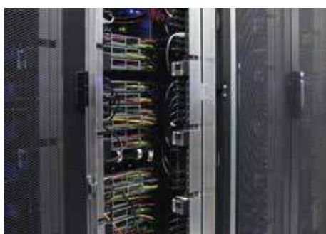
Vertiv™ Knürr® DCM Heavy-Duty Rack server rack for cooling with Liebert DCL, Liebert power distribution modules and integrated cable management
