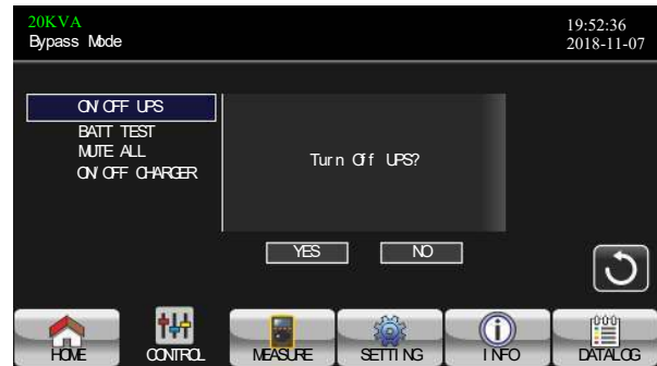
TURN OFF UPS
