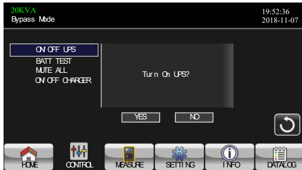
TURN ON UPS
