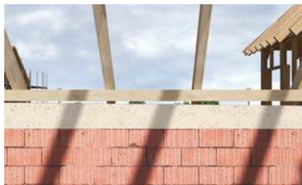
Wooden beams adjustment
