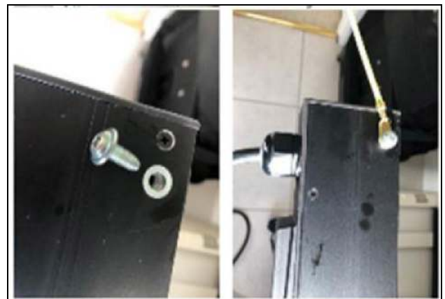
Fig. 15: Housing earthing point of the PDU
