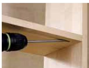
...then you join the two workpieces with wood screws...
