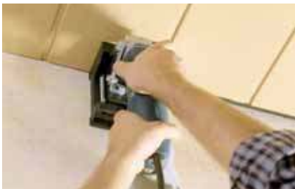
cutting of shadow joints
